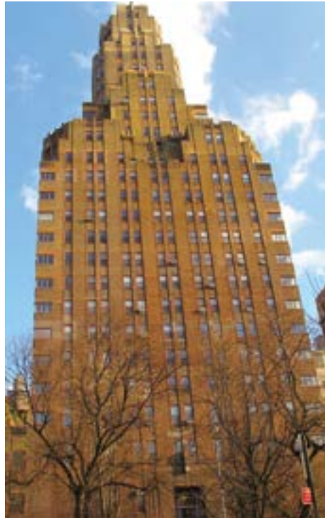
O edifício do Master Institute of United Arts
